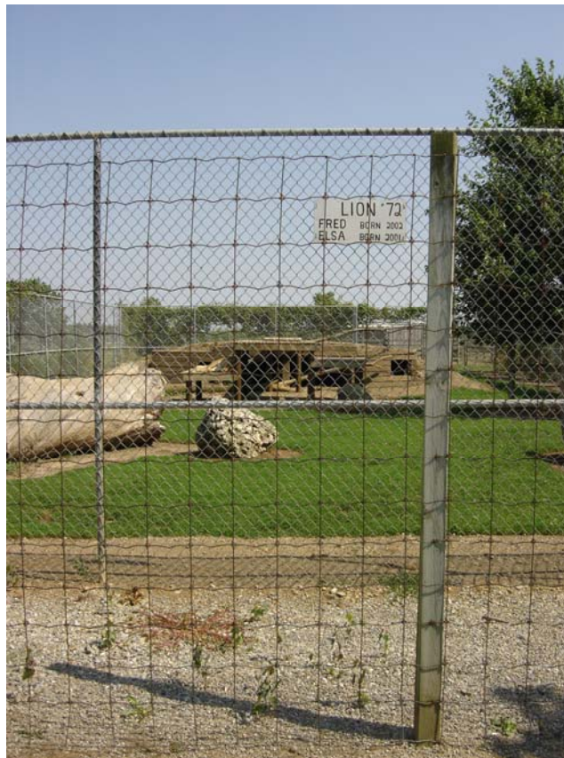
Lion pen fence is very low and not equipped with an inwardly projecting overhang.
