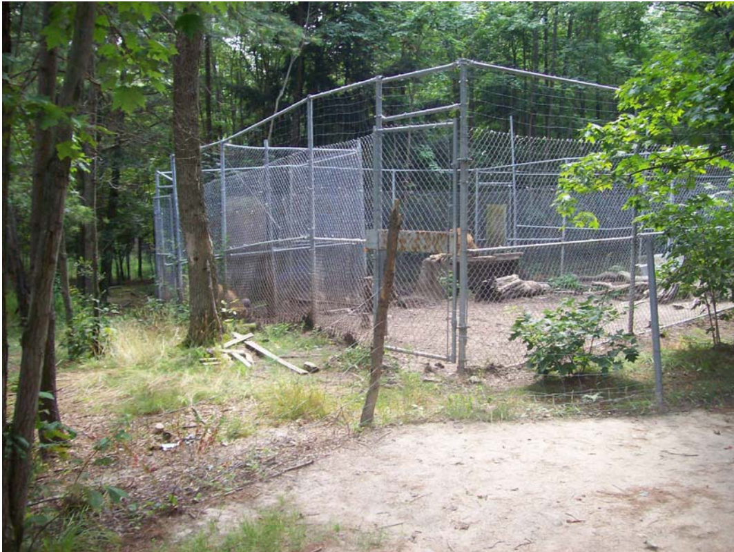
This ramshackle lion cage is small and barren. The fencing is poorly constructed, not equipped with an overhang section at the top and the gate does not properly fit the frame.
