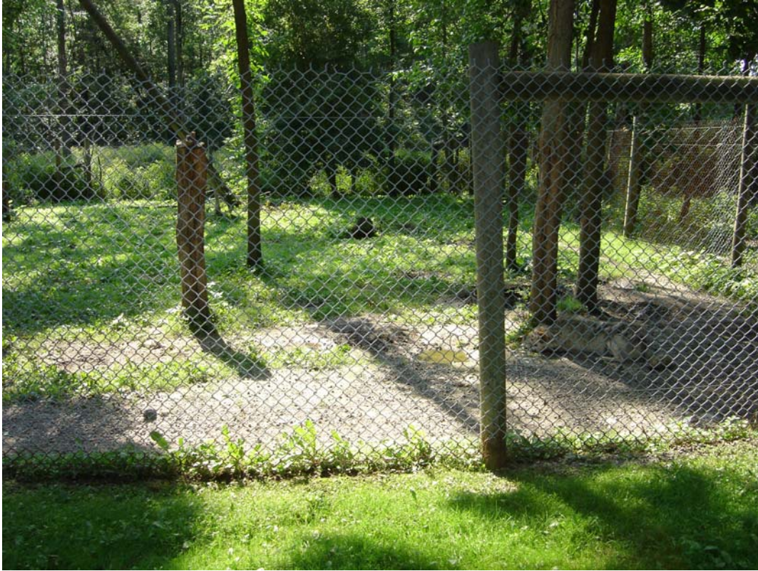
This fence on this wolf enclosure is low and not equipped with an overhang at the top.
