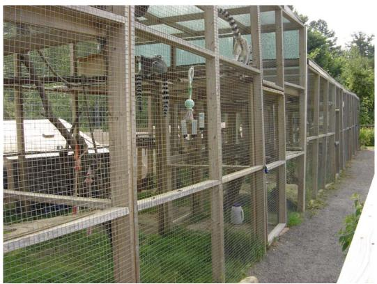
The cages and enclosures are constructed primarily of wooden frames with wire fencing and of very simple design.
