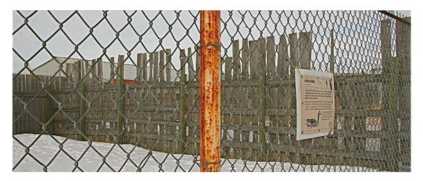
The fencing was in a state of disrepair missing numerous boards and the posts on the chainlink fence are were very rusty.
