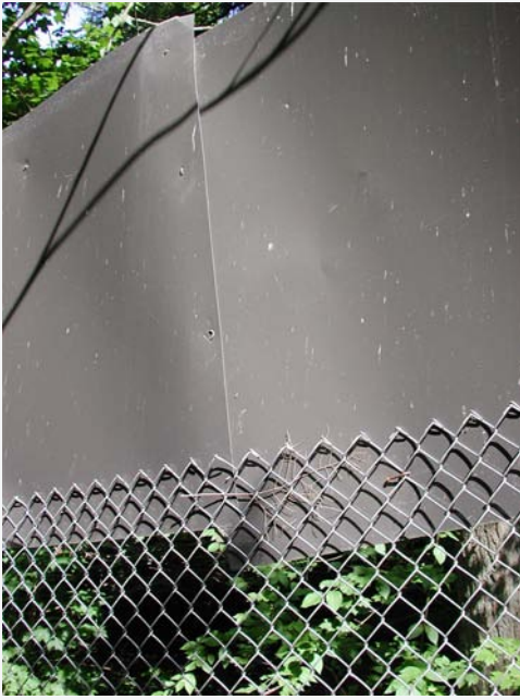
Figure 4. Heavy gauge metal sheeting mounted above chainlink.
